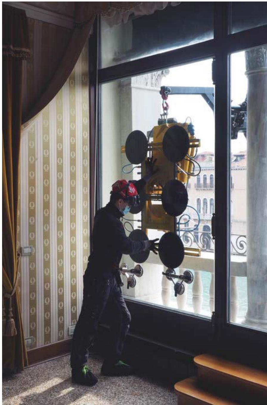
**EN** • Removal of damaged glass and installation of a new armoured set by crane truck mounted on a barge positioned on the Grand Canal.
