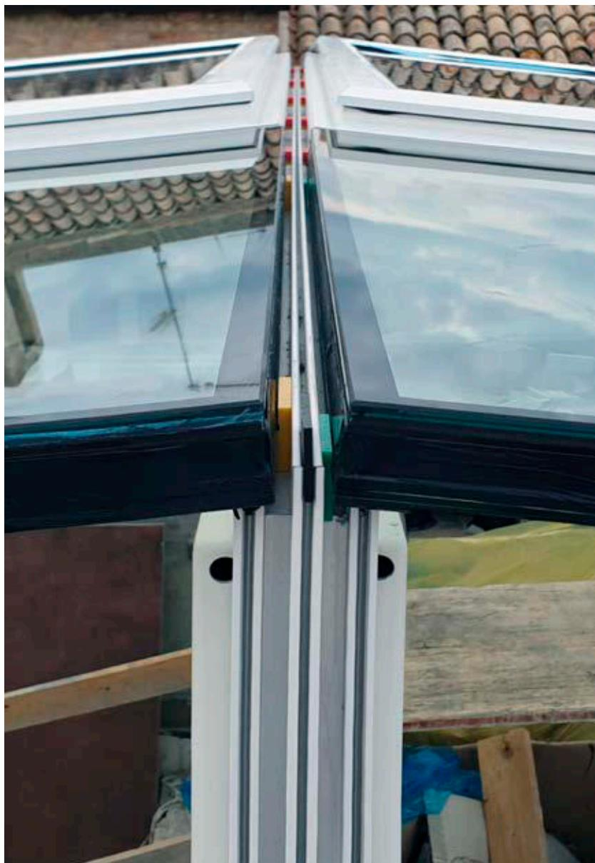
**EN** • The project required particular attention in the design and sizing of glass and frames in order to obtain the effect of external coplanarity.
